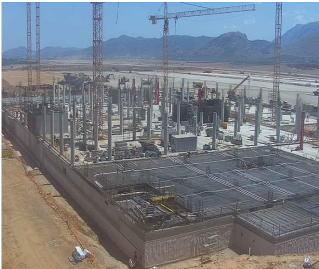
Terminal Building – Columns Concreting
